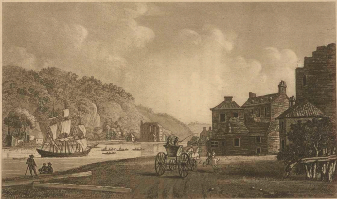
Approach to the Hotwell House.
